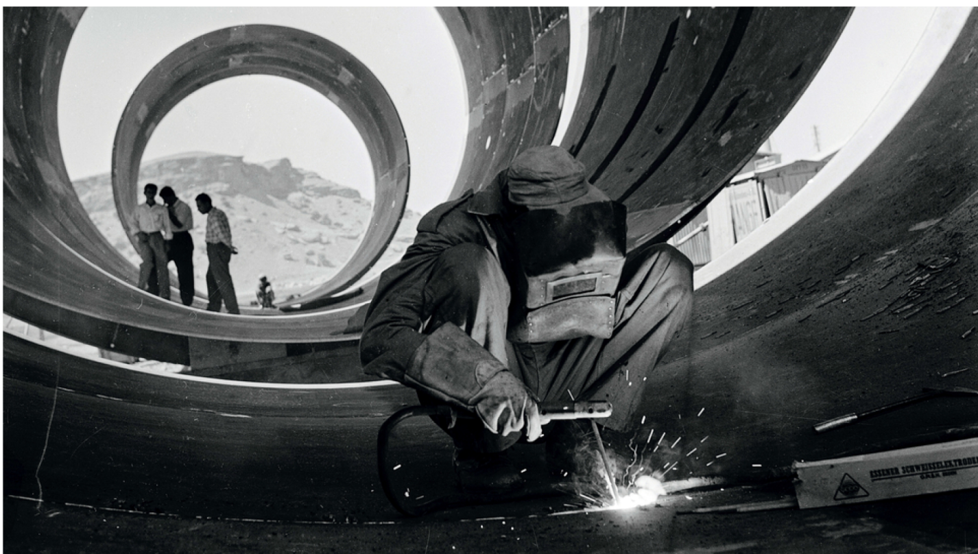
Latif Al-Ani. Building the Darbandikhan Dam. 1961.
